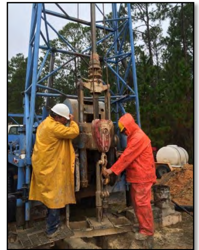
Working on a drill rig in South Carolina.
