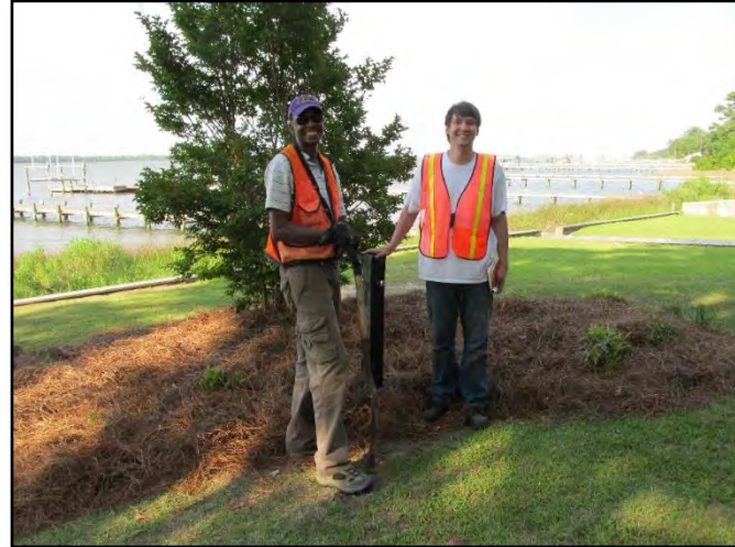
Dr. Alex Manda (left) and James Owers (right) stand next to a newly completed monitoring well.
