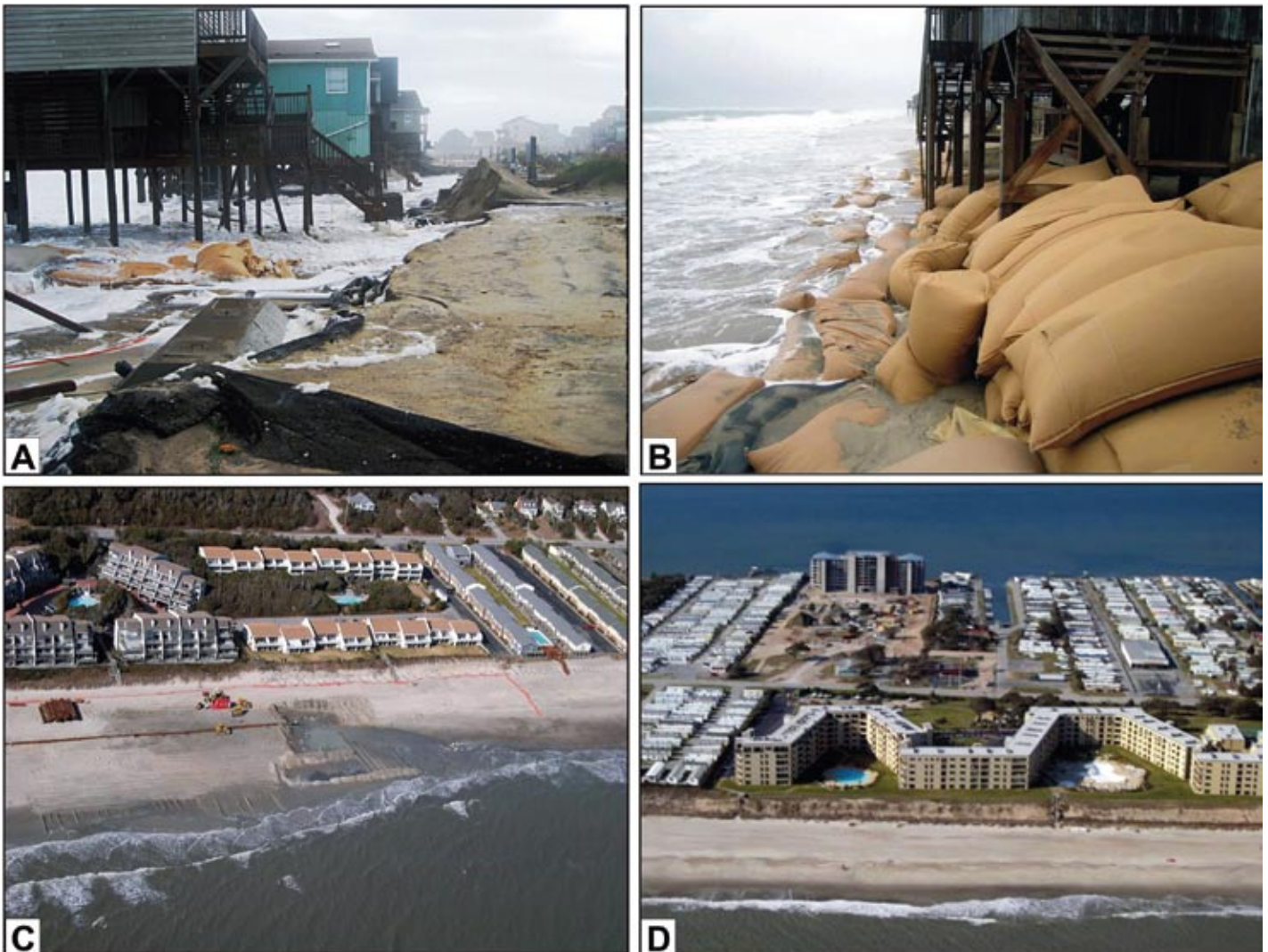
Figure 27. Panel A. A September 25, 2008 photograph shows that the ocean shoreline in South Nags Head has receded so far that sand-bagged houses are now in the surf zone. Septic tanks and associated drain fields are destroyed, the shoreline is actively eroding the access road, and the sand bags have either been moved or sunk into the sand by wave action. Panel B. Photograph shows ocean-side of sandbagged houses in South Nags Head on Bodie Island. Panels C and D show a nearly impenetrable “wall” of structures on Bogue Banks. Moderate storm surges will be funneled between the structures, increasing the risk of flooding and damage to structures further from the ocean front. A very large storm surge may destroy many of the structures, producing large overwash deposits and possibly an inlet if the geologic framework is conducive to inlet development. Photos A and B: ECU/Stan Riggs. Photos C and D: Carteret County Shore Protection Office.
