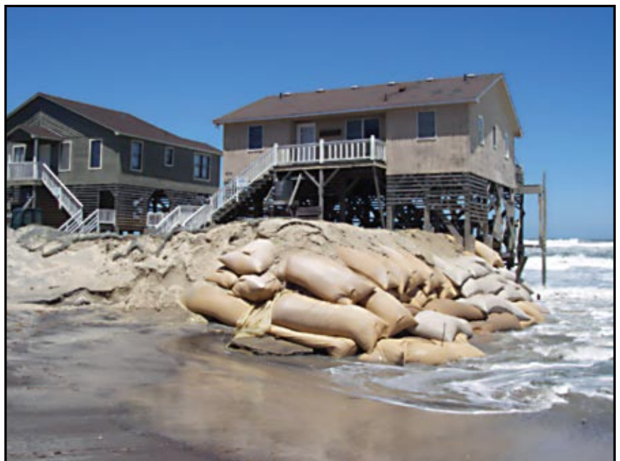
Figure 29. A) The 1998 aerial photograph of a portion of South Nags Head displays the location of the 1849 shoreline (red line) relative to the shoreline location in 1998 (black line). The location of the shoreline is shown in recessional sequence for 1940, 1955, and 1962 (white lines). B) The 2008 photograph shows a house built in the 1980s, encased in sand bags for several decades, and the receding shoreline lapping around the house. The red star indicates the location of the house. Photos A and B: ECU/Stan Riggs.
